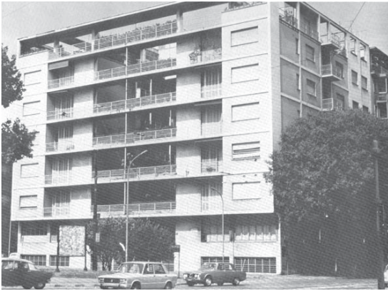
Modern adaptation of traditional Italian courtyard or palazzo building. Two parallel slabs connected by transparent balconies (unifying element).
