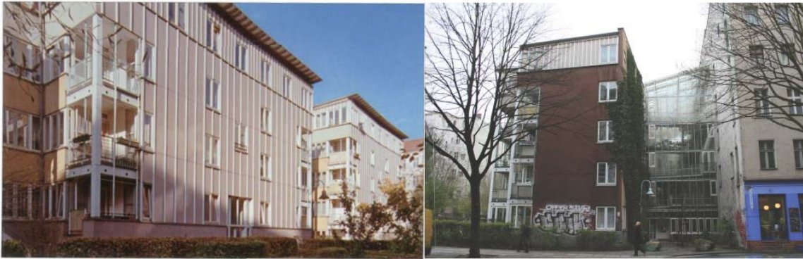
New building; extension of an existing structure (French 177).
