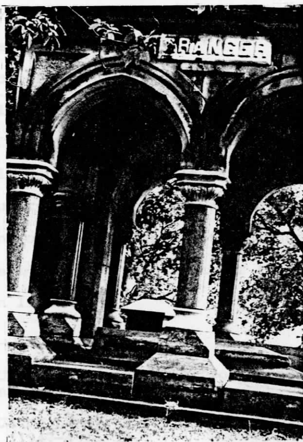
Figure 55 Limestone plinth and granite columns
