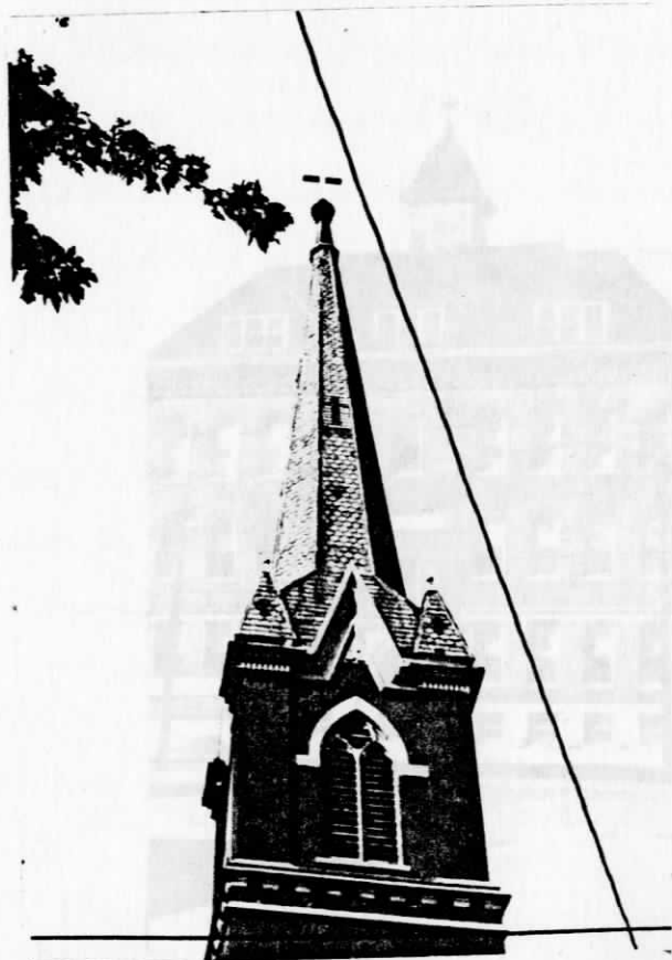
Figure 42 Window in third stage of large tower
