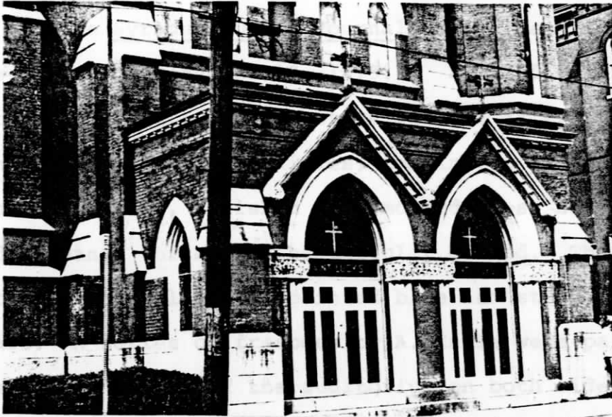
Figure 43 Main entrance, south facade
