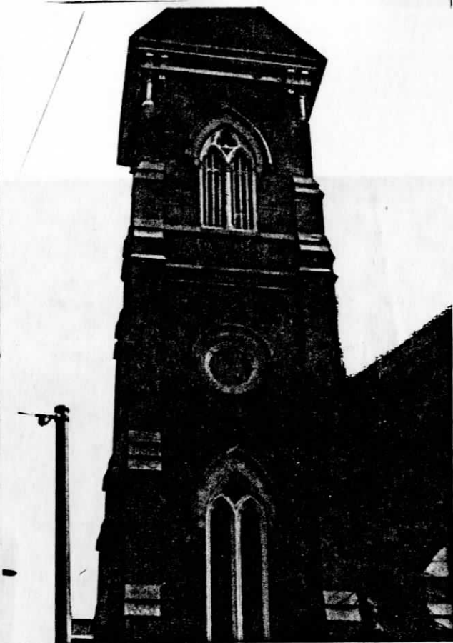
Figure 38 Lancet window with corbeled dripstone
