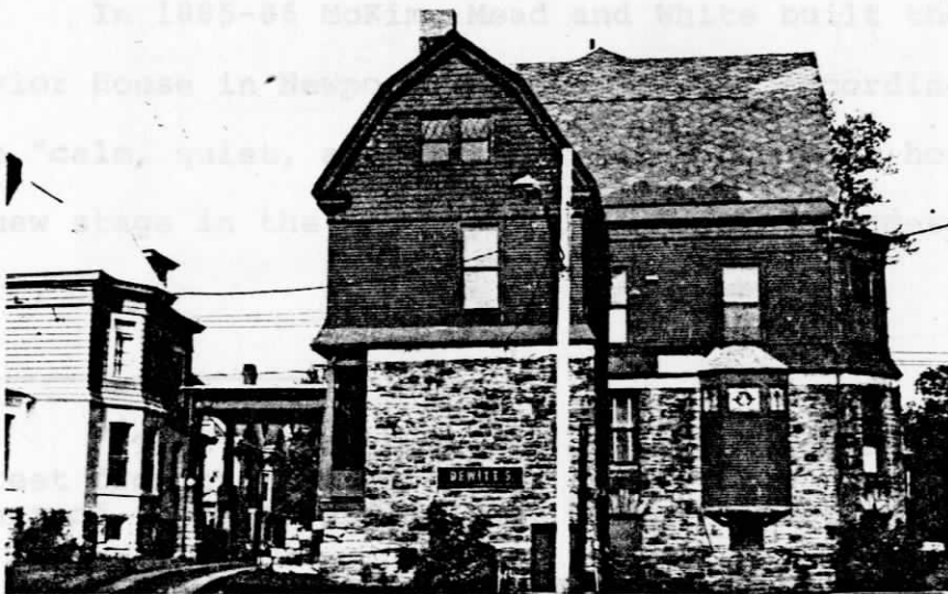
Figure 90 Polygonal bay, south facade
