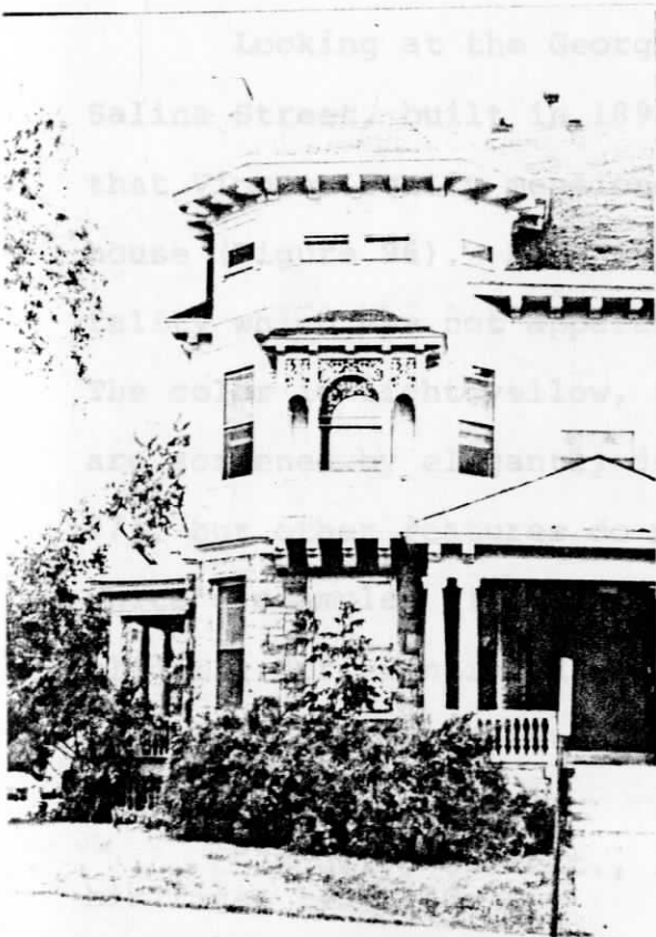
Figure 93 East facade with projecting pavilion and porch
