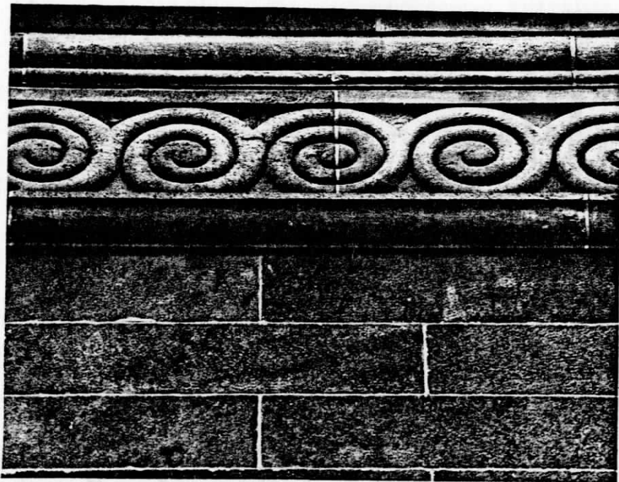
Figure 28 Circular spiral motif on east facade
