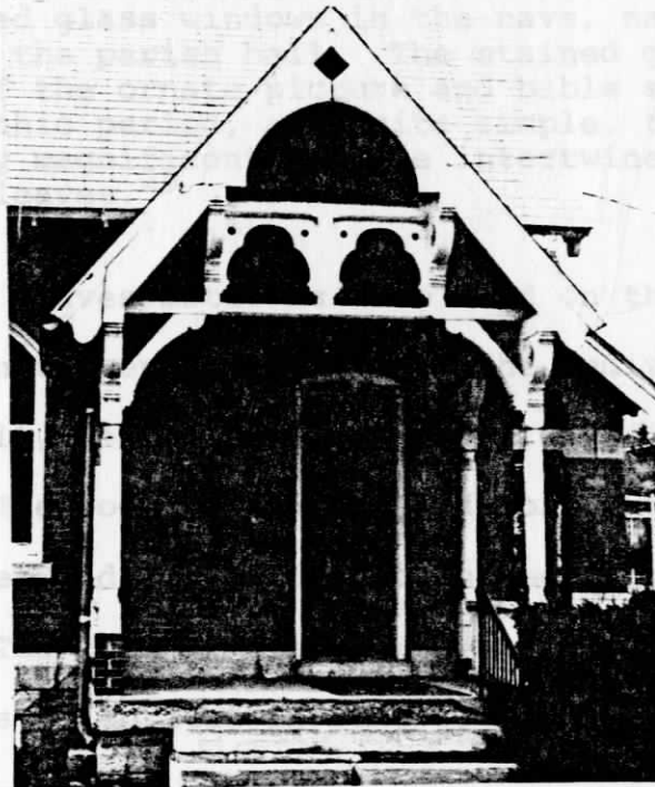
Figure 51 Porch on east facade
