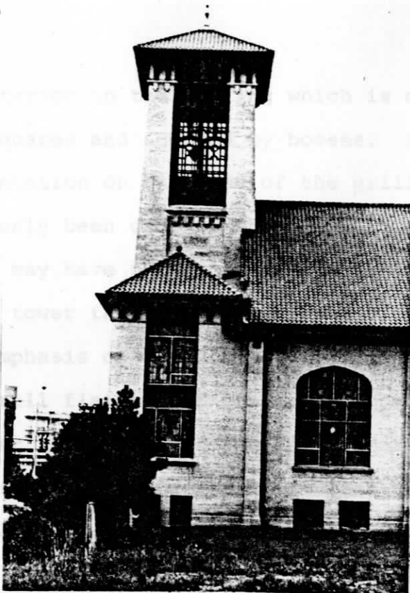
Figure 123 Projecting piers and carved stone dentils on east facade
