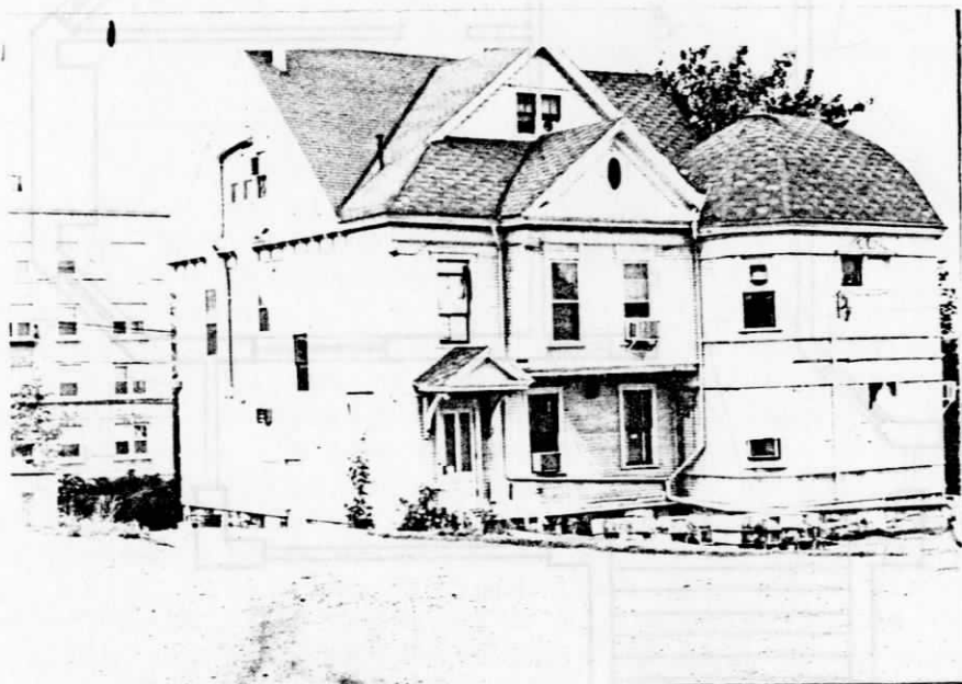
Figure 86 Variegated roofing, north facade
