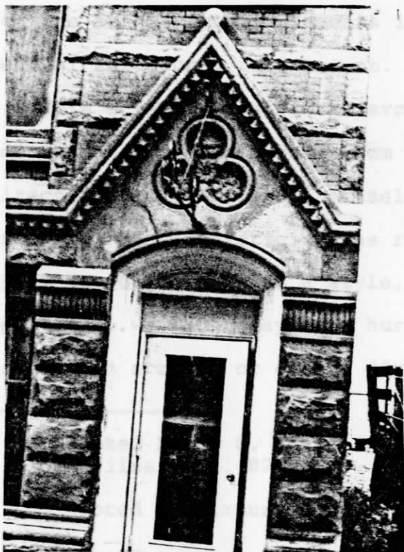
Figure 118 Side door on south facade
