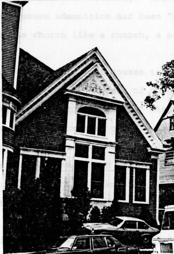
Figure 76 Aedicule window on south facade and projecting entablature
