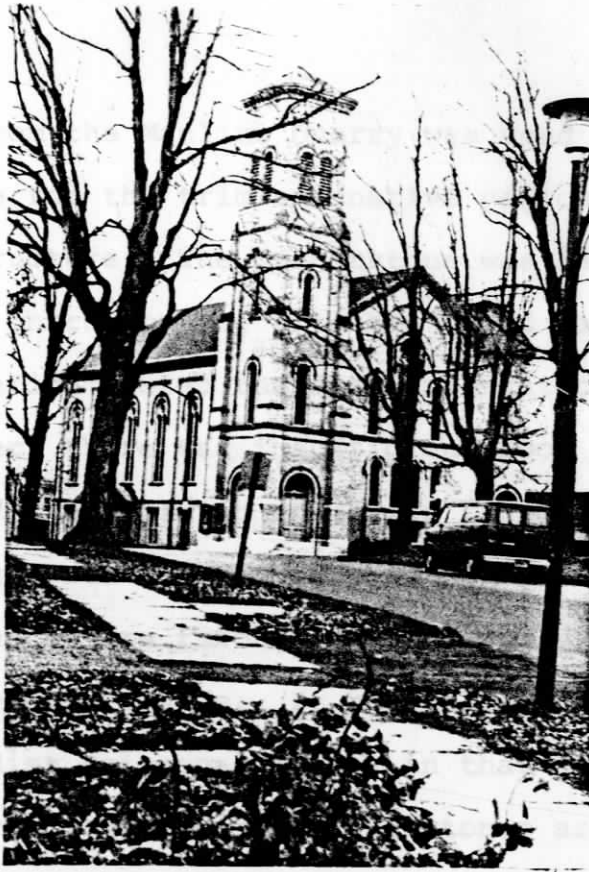
Figure 4 Cazenovia Methodist Church (1872) Linklaen Street, Cazenovia, N.Y.
