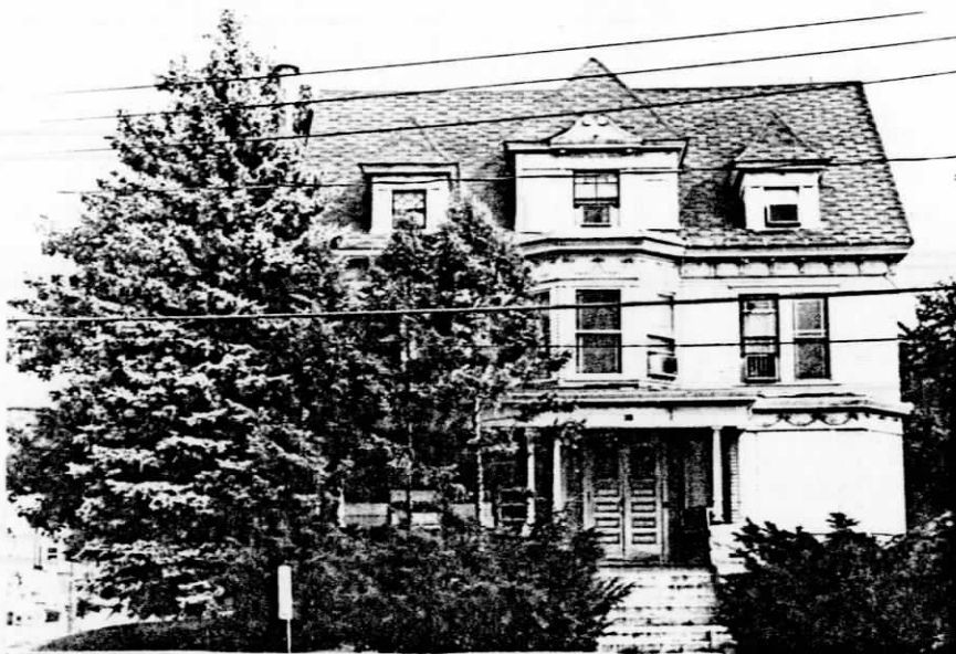
Figure 85 Charles F. Ayling House (1893) 601 University Avenue and Harrison Streets Syracuse, N.Y.
