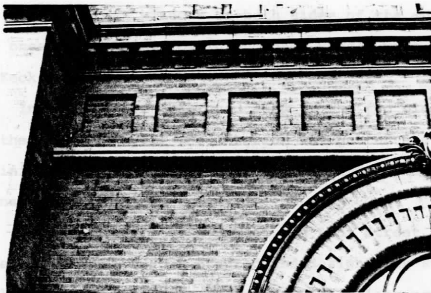
Figure 10 Beltcourse and archivolt molding, south facade
