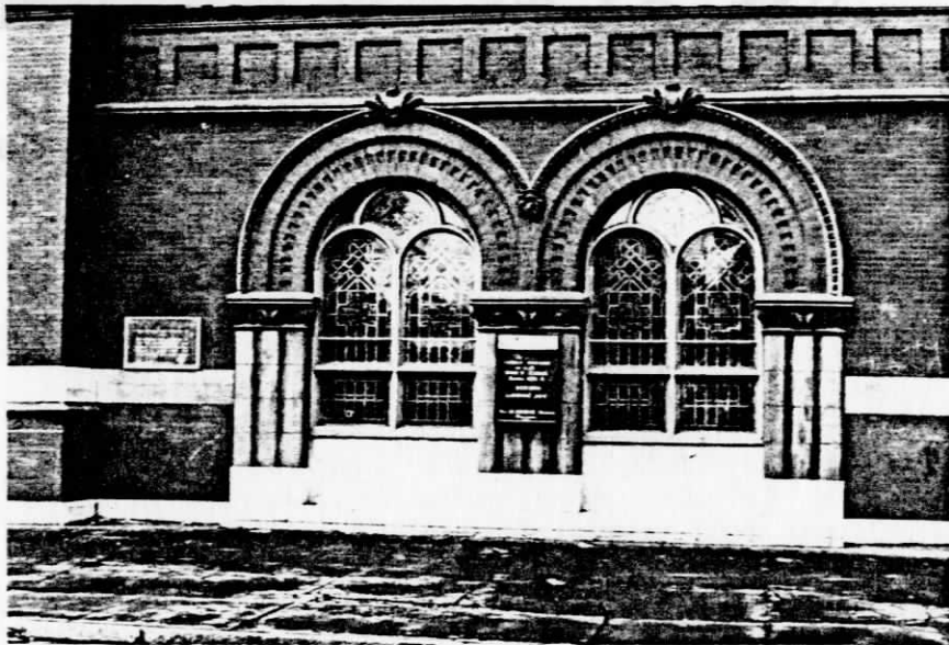
Figure 9 Former Entrance on Delaware Street
