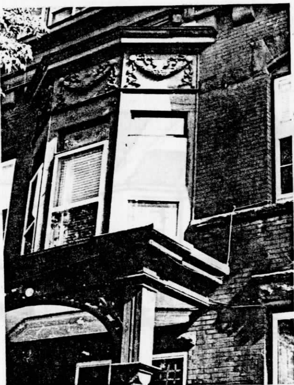
Figure 84 Bay window on east facade
