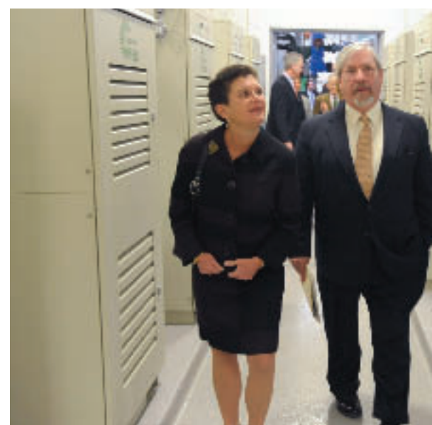
Above: SU Chancellor Nancy Cantor and Francis J. Murray, president and chief executive officer of NYSERDA, tour the green data center facilities, touted to use 50 percent less energy than a typical data center.
