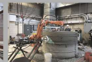
Figure 5 Concrete Printing https://news.psu.edu/story/583678/2019/08/13/research/research-team-receives-grant-commercialize-3d-printed-concrete
