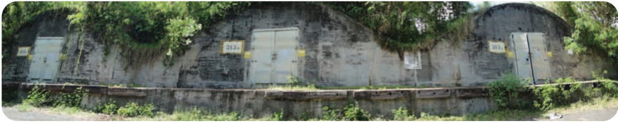
Bunkers. They served as ammunition storage. These bunkers are covered with local flora.
