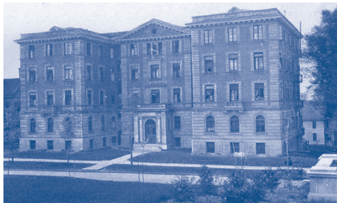
Original Haven Hall
