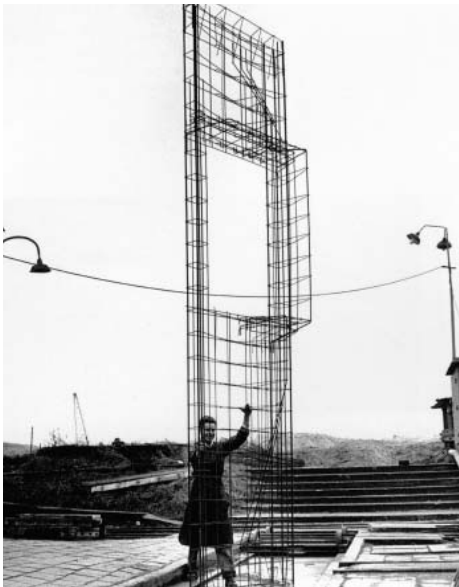
At left, the initial design for Robinson House, December 1946 (left). Above, the reinforcement for facade element to be cast in concrete, Nivelles, Belgium, 1963-64.
